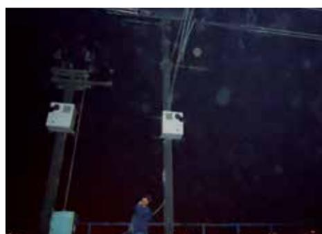
The FLIR E50 thermal imaging camera is installed in an IP66 rated enclosure.
